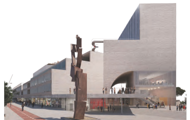
View of the Business Center from Syntrivani Square
