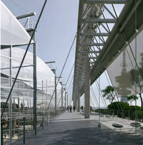
View from level +1 of the gallery on the Exhibition Center side
